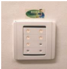
“Save Energy” stickers on the switch panel
