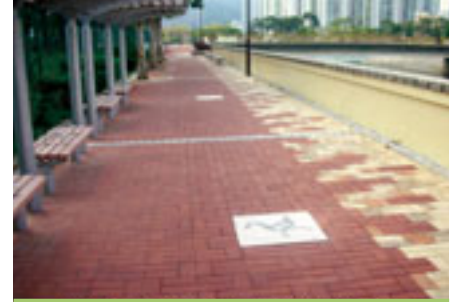
Paving block designs with 2008 Olympic and Paralympic Equestrian Events pictograms were embedded in pavements.
