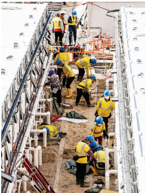
Working with contractors throughout challenging times.
