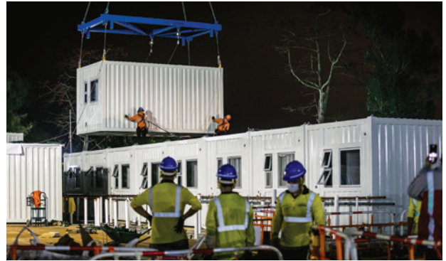
Construction and installation of MiC.
