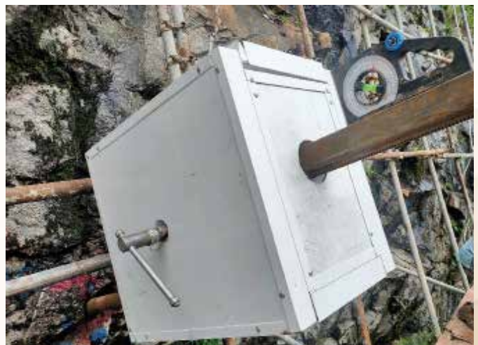
To better achieve noise reduction effect, the project team installed a tailor-made sound insulation box on the outer side of the motor.
